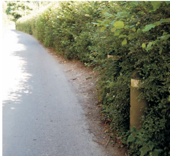
Careful siting of bollards to prevent over running and aid hedge recovery
