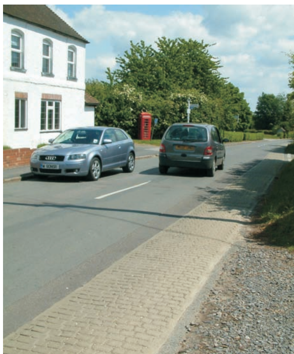
Alternative provision for pedestrians through a village
