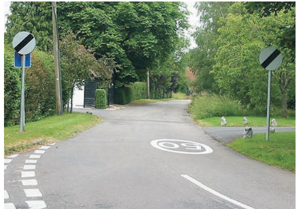
Where mandatory signs are required, co-location should be considered to reduce sign clutter
