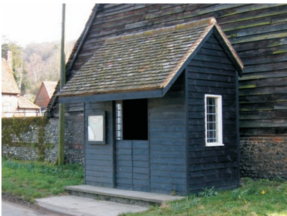
Use of vernacular materials and styles will help bus shelters and other structures fit into the local setting
