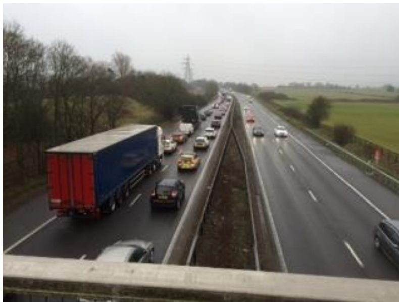
A1 (M) South (from other side of the bridge) 09.05 a.m. - 1 March 2016
