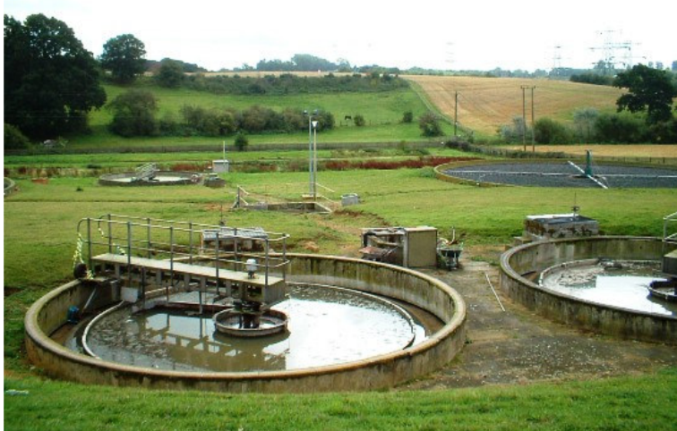
Figure 7-35 Existing settlement tank at Ashbrook WwTW
