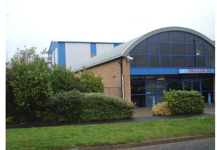
2. Warehouses are made of corrugated iron and brick. Wide verges can lighten up the industrial landscape.
