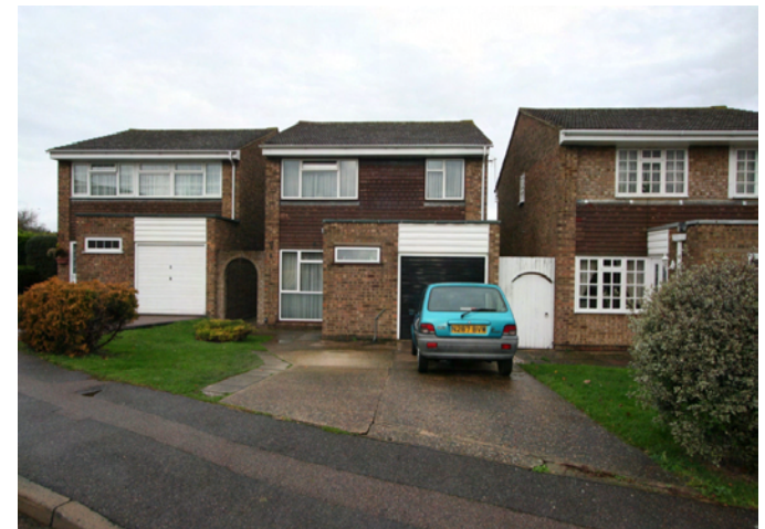
8. Single-design units in the Post-war Suburban Zone, using brown brick, wood cladding, roofed with concrete tiles.
