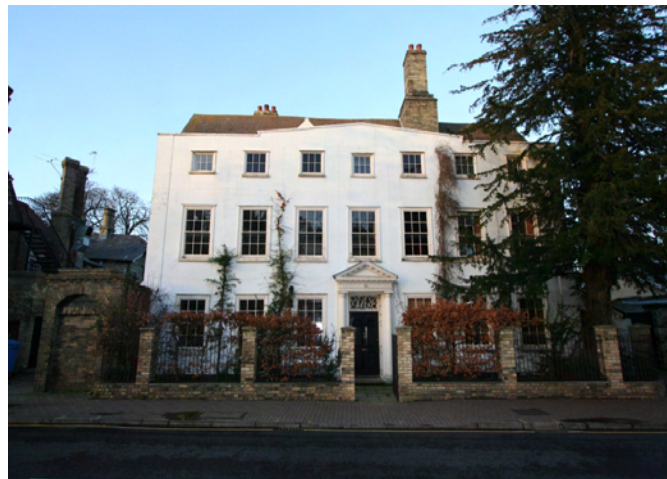
3. The finely proportioned and subtly pedimented classical render at 18 Melbourn Street (Grade I listed).
