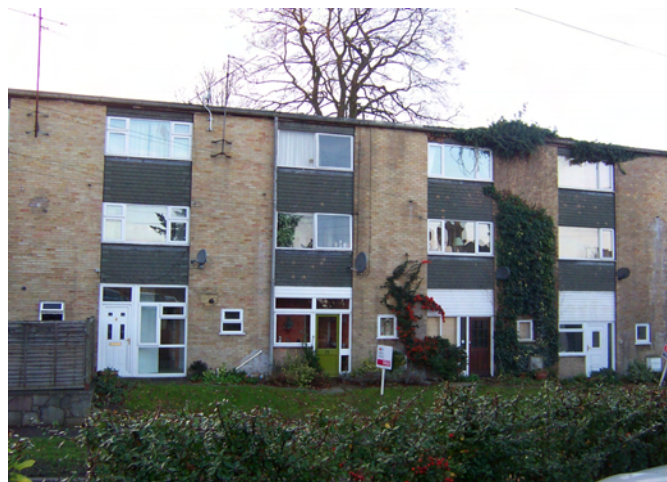
7. A block of flats in the Post-war Suburban Zone.
