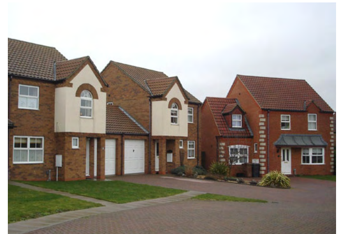
4. High densities in the new Fieldfare Way estate.
