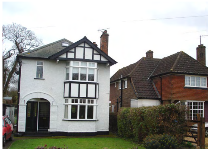
7. Inter-war brick detached house with curved porch, timberframe rendered gable and bay window, neighbouring a post-war house in Green Drift (Low Density Mixed Residential Zone).
