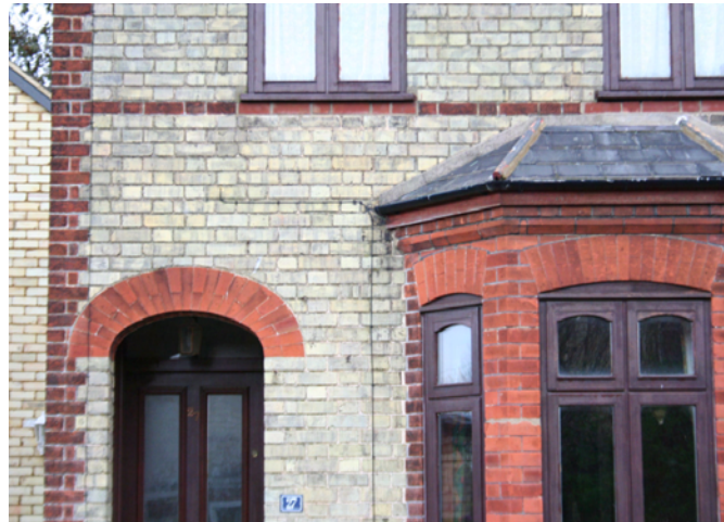
5. Victorian yellow brick housing, with red brick bay windows and decorated porch on Morton Street, (Historic High Density Zone).
