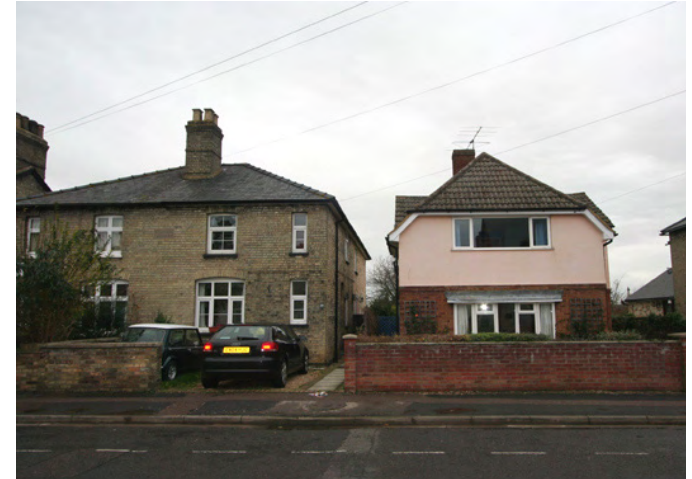
2. High densities in the Historic High Density Zone, reduced by lower density infill.
