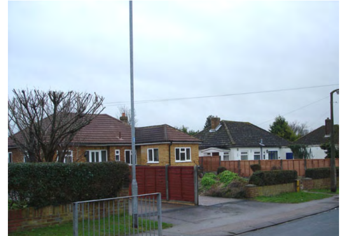
6. Wide but regular gaps at Serby Avenue.
