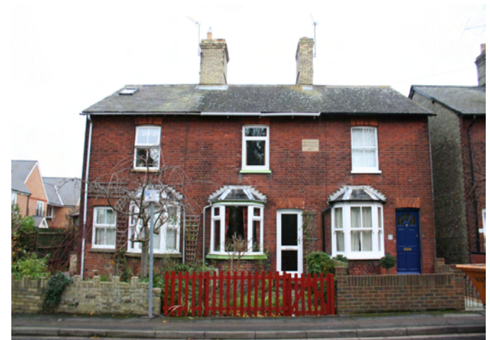
4. Red brick Victorian terraces.
