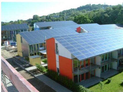
Fig 6: Use of photovoltaics on roofs in Freiberg, Germany (Alex Ely: CABE)
