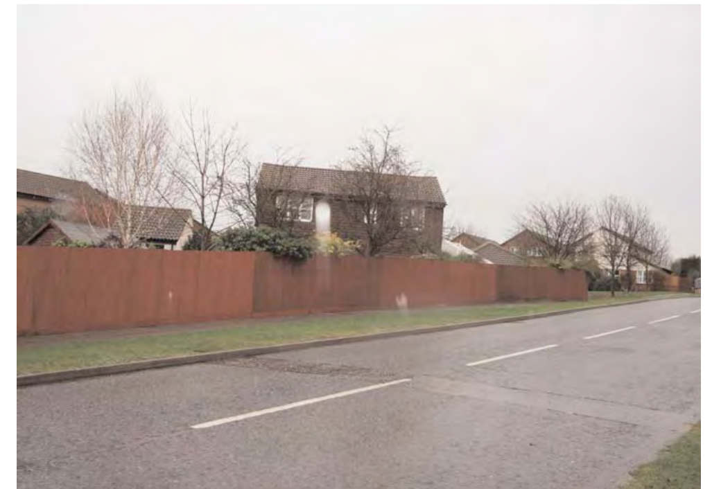
4. The blank frontage created by the backs of properties means a lack of natural surveillance along these key routes.
