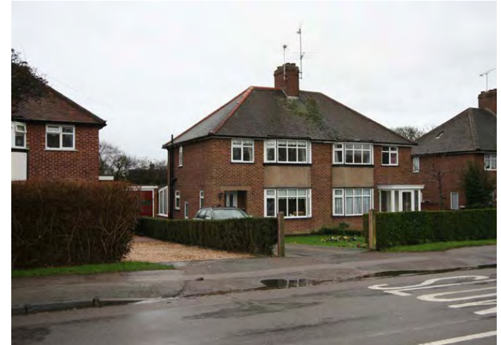
2. The quality of paving varies within the Interwar/1950s areas with ad hoc repairs in differing materials and colours.
