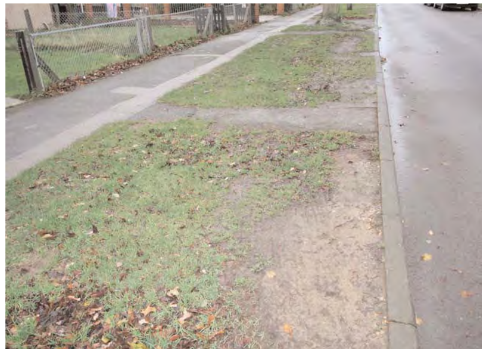
1. Damaged grass verges due to the lack of parking within the Monklands residential area part of the Garden City zone.
