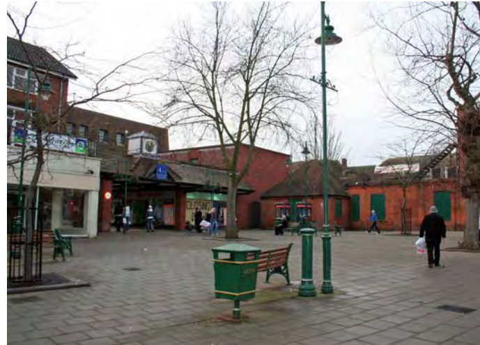
1. Leys Square is an important public space in the town centre although it is poorly fronted on two sides.
