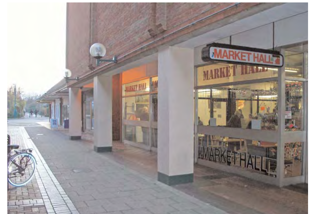
4. The poor quality of the Market Hall is seen to project a negative image of the town centre.
