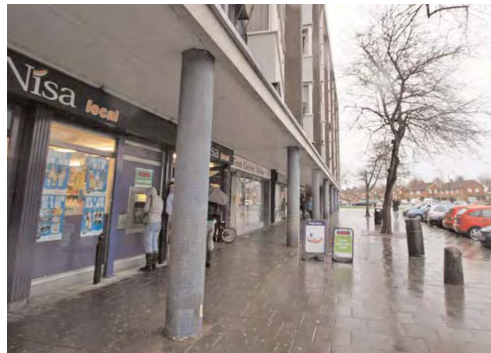
3. One of the small local retail parades in the Grange Estate within the Postwar residential areas.
