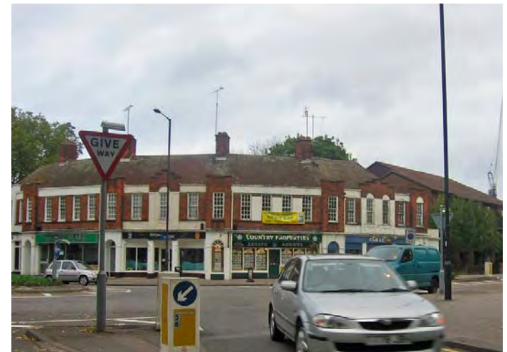
4. More domestically scaled buildings at the edge of the town centre.
