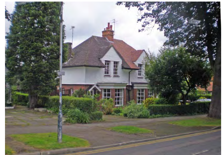
4. Within the Garden City residential area some pavements have been damaged, and grass verges have been lost where parking pressures are high.
