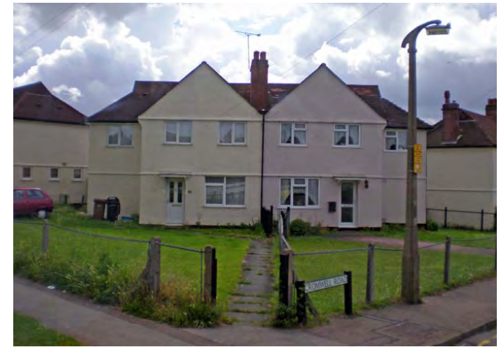
2. Special attention was paid to corner plots where buildings were often positioned at an angle within the plot within the Garden City zone.
