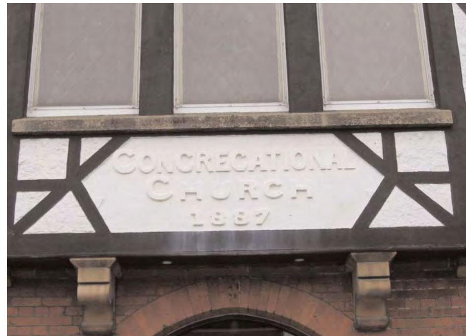
1. Detailing at the Congregational Church on Station Road provides a visual link with the past.
