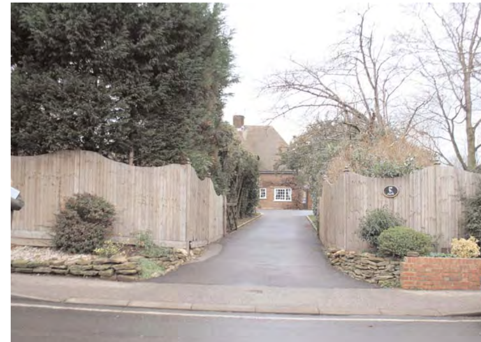
2. Properties set within large plots with very large setbacks along Park Lane within the Semi-rural Zone.
