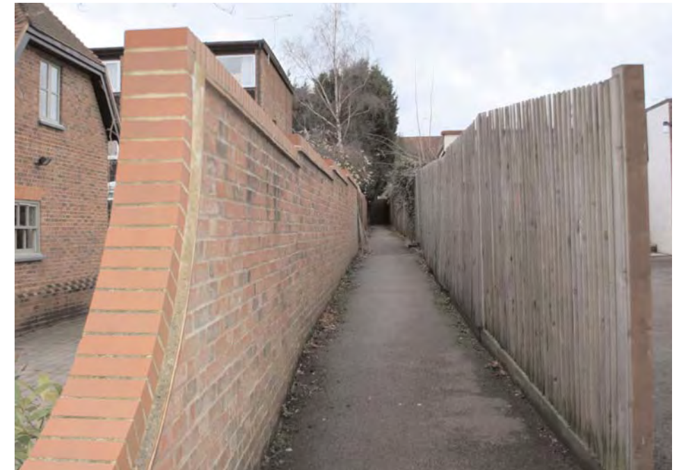
2. Poorly lit pedestrian footpath along Westland Road within the Postwar Suburban area.
