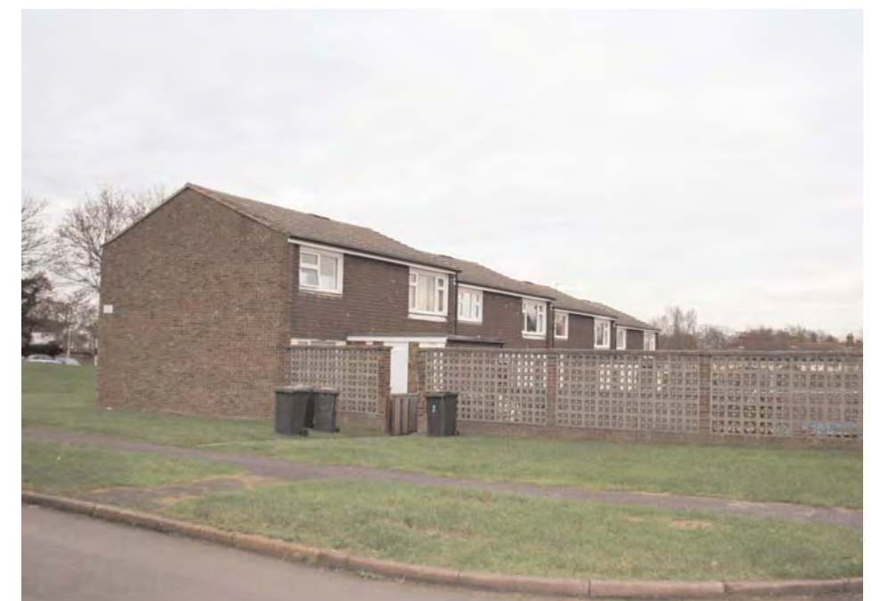
4. Blank facades to the street created at corner plots within the Postwar Suburban area.
