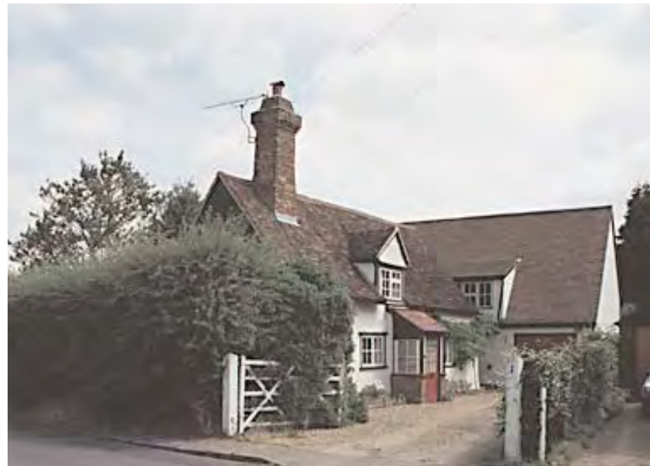
3. Grade II Listed 18th century cottage at Gun Lane
