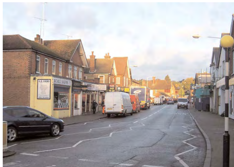
3. The building line along both sides of London Road is fairly consistent to the pavement edge.
