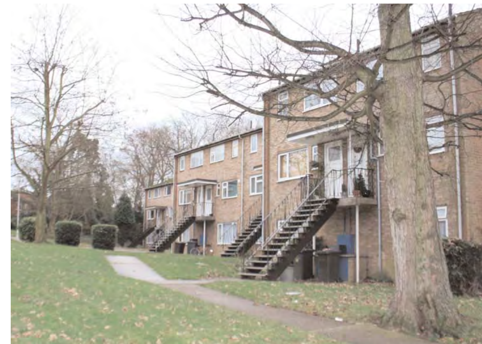
3. Three storey maisonettes along Haygarth within the Postwar Suburban area.
