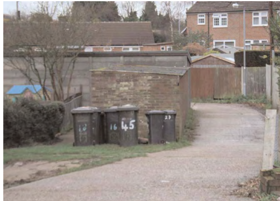
1. Garage court off Deanscroft; the lack of natural surveillance from surrounding properties of these areas means that they tend to attract anti-social behaviour.
