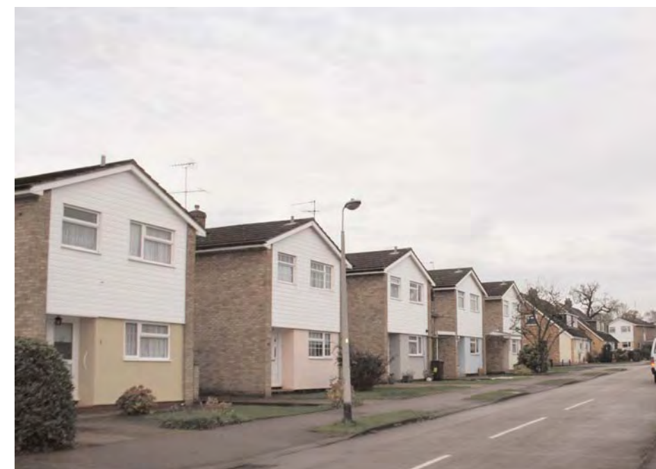
4. A row of detached houses parallel to the road with continuous building line and small setbacks along Sayer Way within the Postwar Suburban area.
