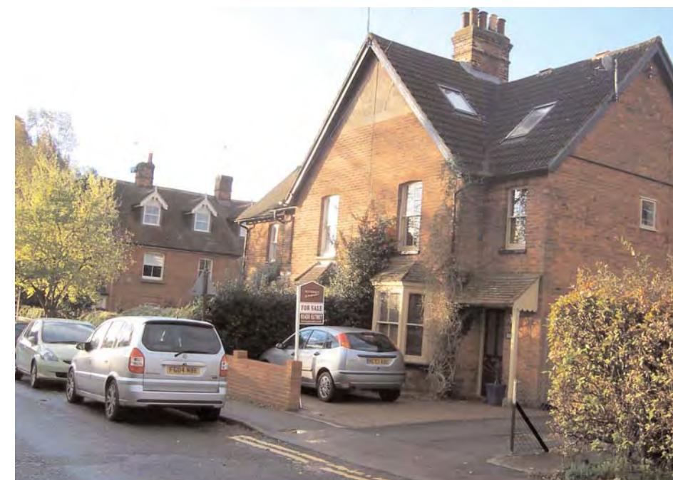
4. Victorian red brick property with gable, hipped and steeply pitched tiled roof and brick chimney along Pondcroft Road within the Historic Inner Zone. The property to the left has dormer windows.
