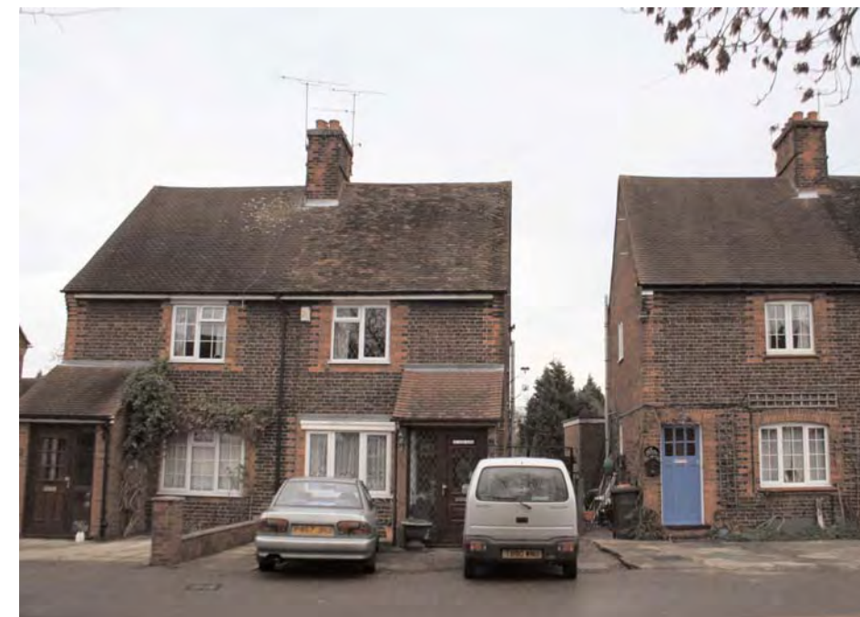
2. Closely spaced terraces with small front gardens, long narrow rear gardens gives a medium to high density character to the Historic Inner Zone.
