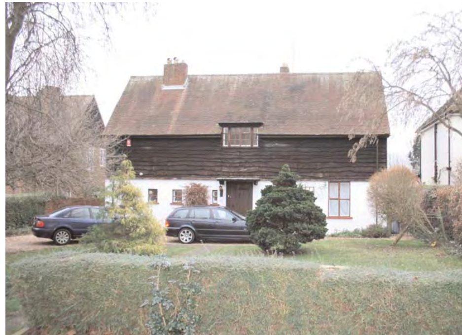
1. Peter's Way - low ground floor cottage windows and weatherboard gables characteristic of Lutyens' early style within the Semi-rural Zone.
