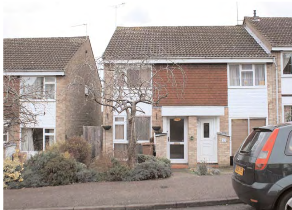
3. Brick construction with timber panelling and plastic cladding on 1970s semi-detached houses at Gipsy Lane within the Postwar Suburban Zone.
