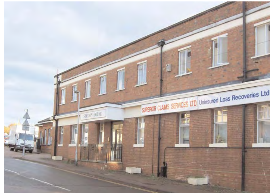
1. Office block adjacent to the station within the Village Centre.
