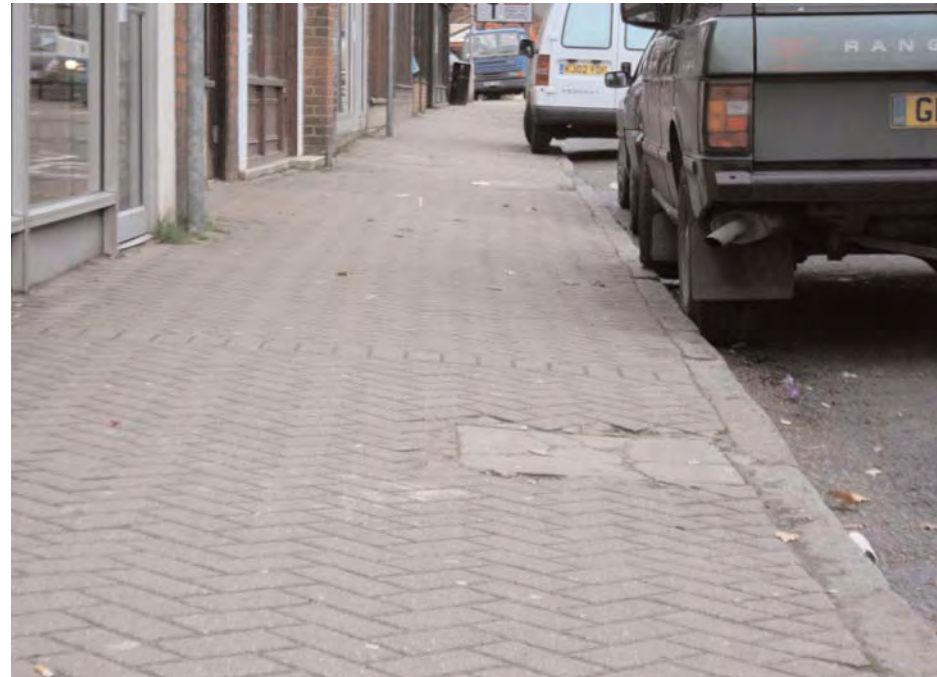
1. Herringbone paving on London Road in the Village Centre.
