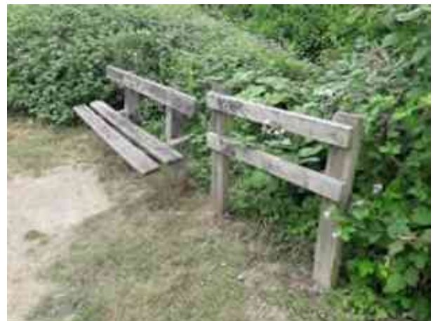
Bench to be replaced
