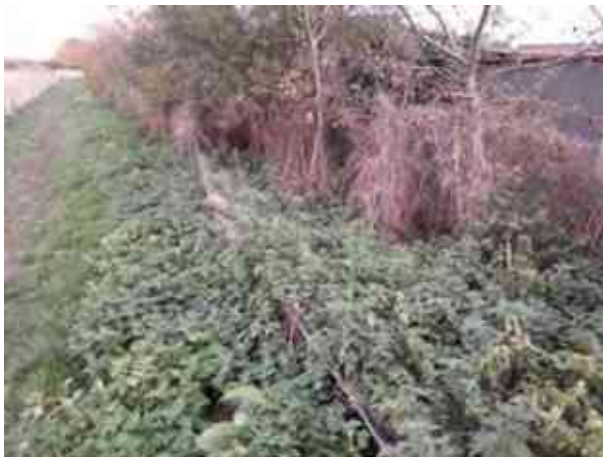
Broken post and wire fence
