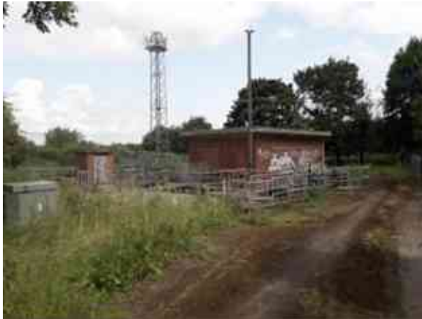
Anglian Water site
