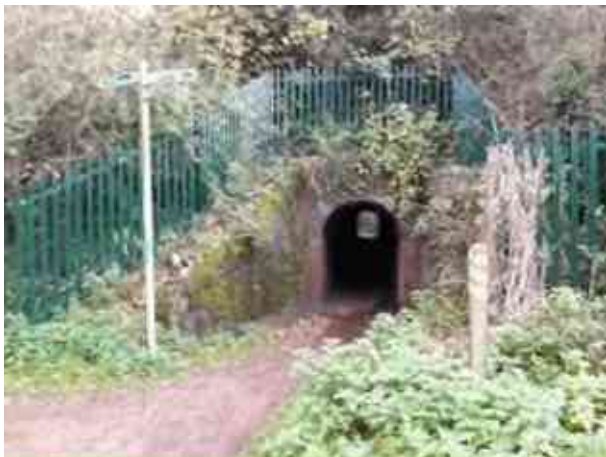
Pedestrian tunnel under railway
