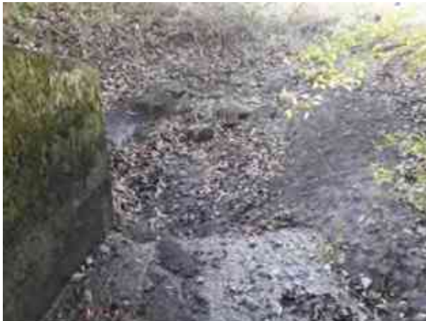
Erosion at Anglian Water site outflow
