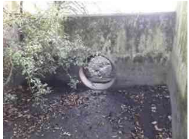
Outflow from Anglian Water site in to wetland
