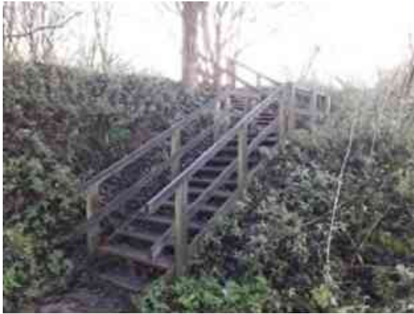
Ladder steps at northern entrance
