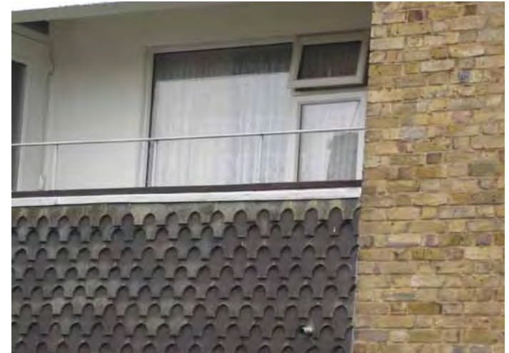
10. Brown brick and tile cladding on a block of flats in the Post-war Suburban zone.
