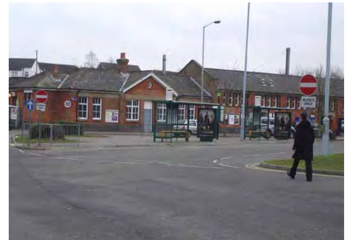
4. The station is an increasingly important gateway to Hitchin, and an improvement to Station Approach could have a large impact on visitor and resident perceptions of Hitchin.
