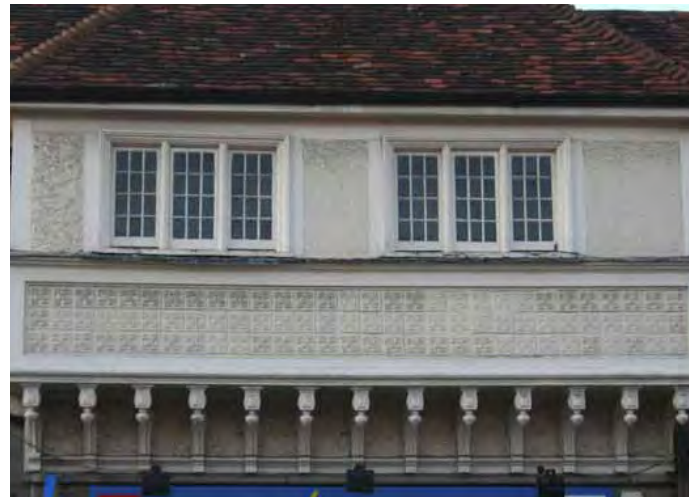
1. Elegantly decorated eaves supporting a projected first floor, common among timber framed houses in the Town Centre zone.
