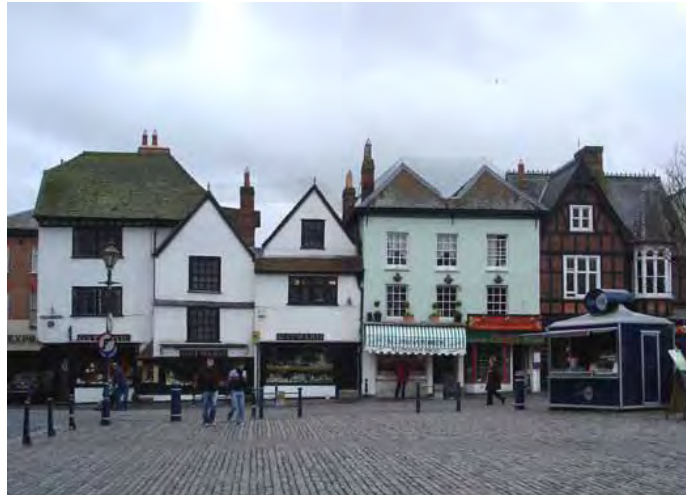
1. Town houses of various sizes form a continuous frontage in Market Square.
