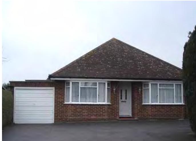
9. A bungalow on Meadow Way built of brown brick with a concrete-tiled hipped roof.
