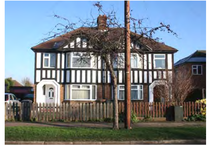
6. Timberframe render with brick ground floor and recessed porches - typical details of inter-war semi-detached houses.
