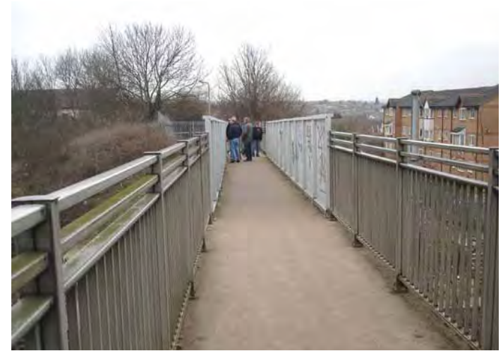
6. The footbridge over the railway is one of only three ways across the railway which forms a barrier right through the western side of Hitchin.
