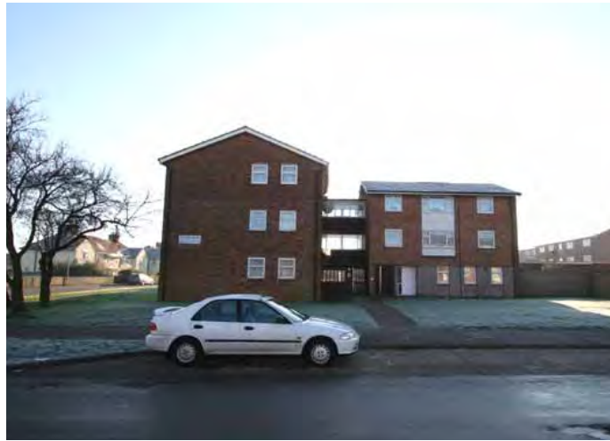
5. Buildings set square to the roadside can offer less active frontages, but open plan gardens allow free interplay between the frontage and the street (Post-war Suburban zone).
