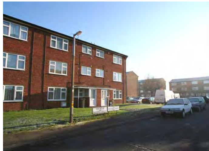
7. Three-storey blocks of flats at John Barker Place.
