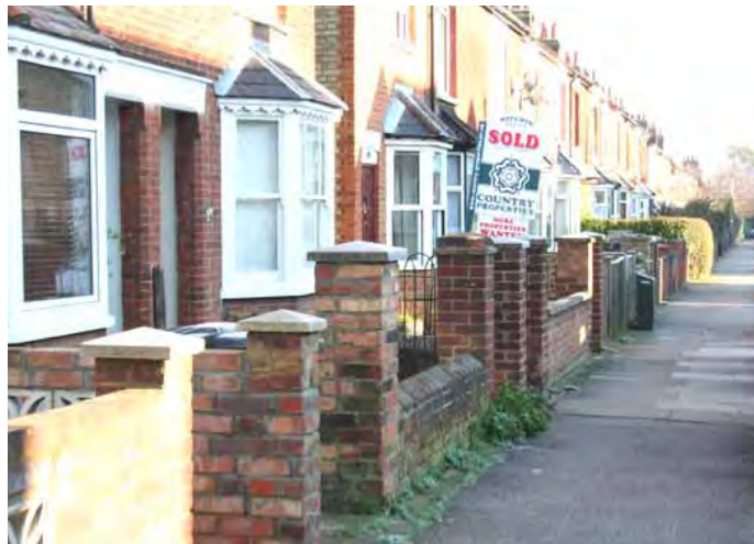
3. Victorian terraced houses on Lancaster Road, Historic High Density zone.
