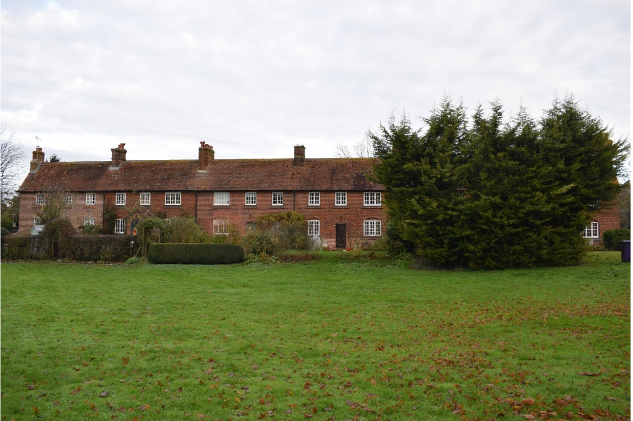
Fig 2.4 Manor Cottages (NLE 1175728) on the north edge of the village green.
