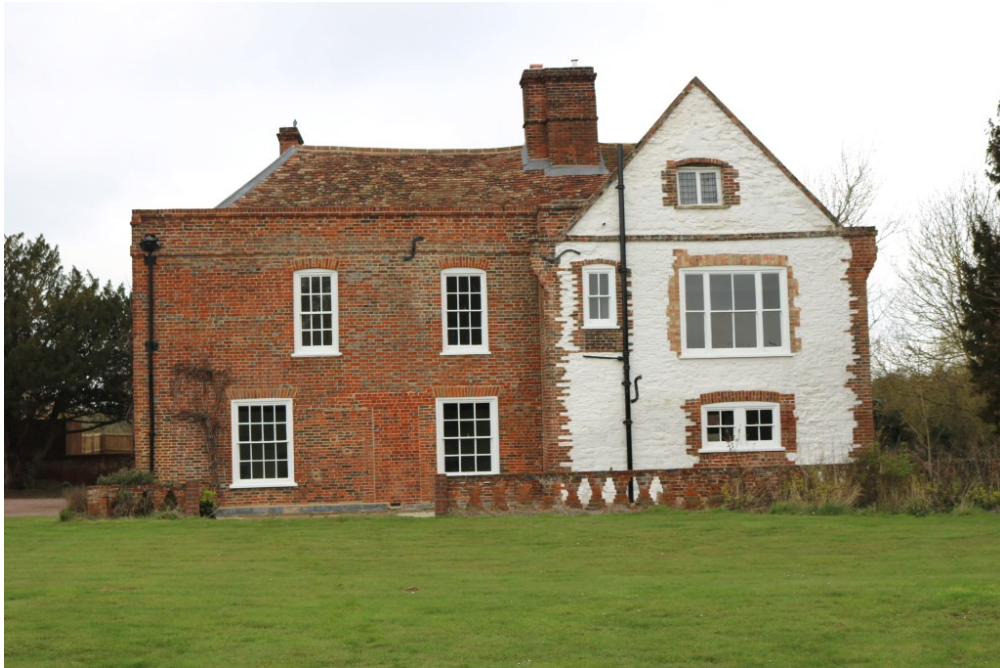
Plate 3: East elevation of the house showing the clunch masonry facing of the 16 th century north-east wing
