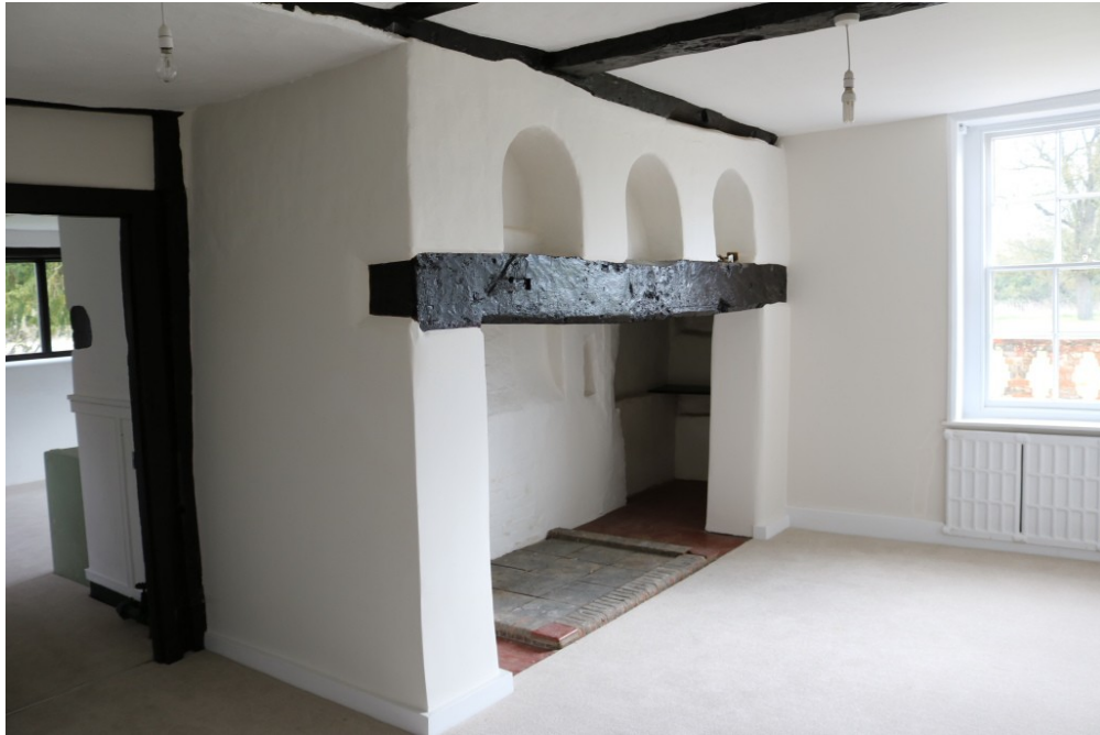
Plate 7: View of the late 16 th century fireplace in the east wing, with three round-headed niches above a chamfered lintel
