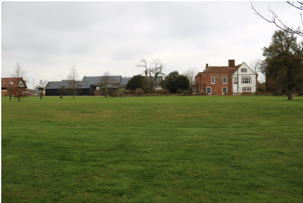
Plate 11: View looking west towards the listed building from within its immediate curtilage land, showing how the presence of former agricultural buildings (currently undergoing residential conversion) restricts views towards the agricultural land to the west
