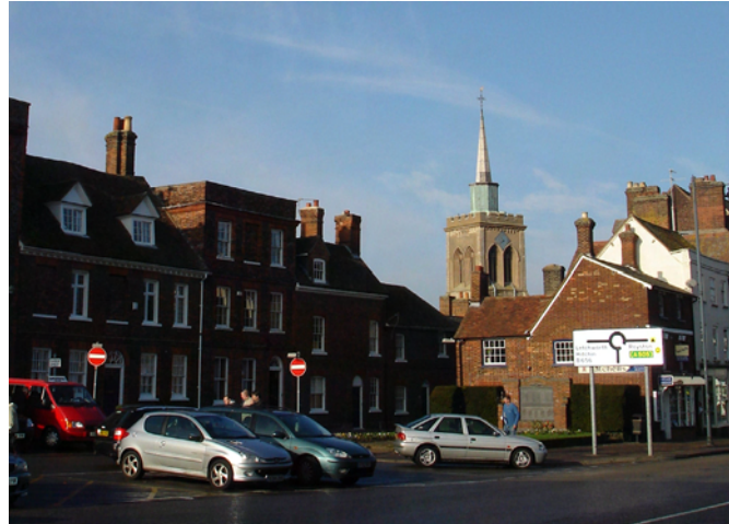
1. Views of St Mary's Church create a visual connection between the centre and the outskirts, aiding the cohesion of the town as a whole.
