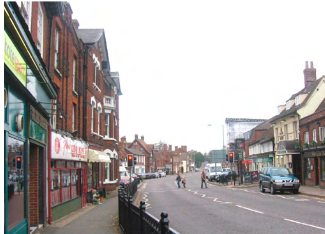
1. Narrow pavements create a car-dominant feel in the Town Centre zone.
