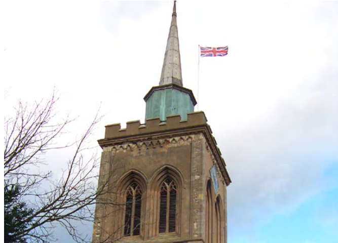
1. St Mary's Church is a very prominent landmark in Baldock as a result of the town's consistent (mainly) two-storey building heights.
