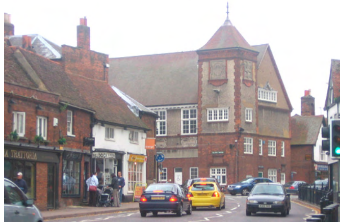
1. The Town Centre zone is geared to traffic flow. The pedestrian environment could be enhanced.
