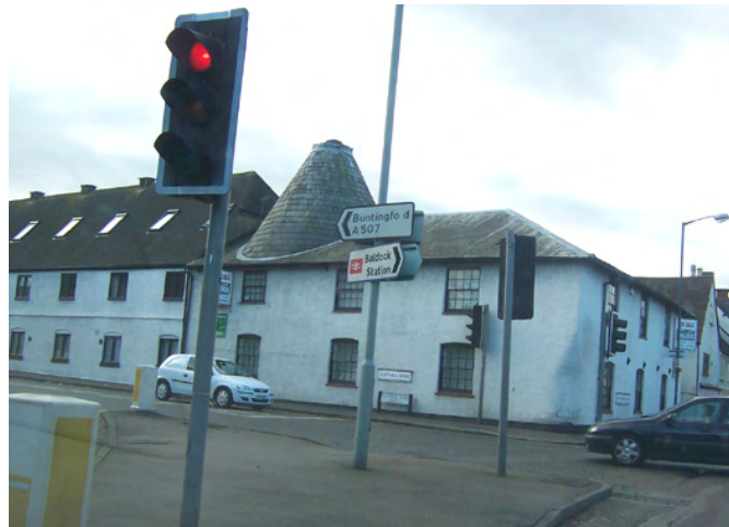
1. There is little soft landscaping in the Town Centre zone in general.
