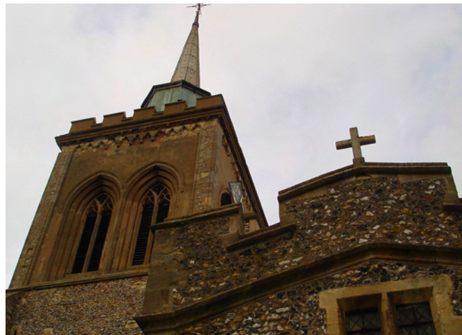
3. Traditional stonework stone and flint at St Mary's Church and the 'Hertfordshire spike'.
