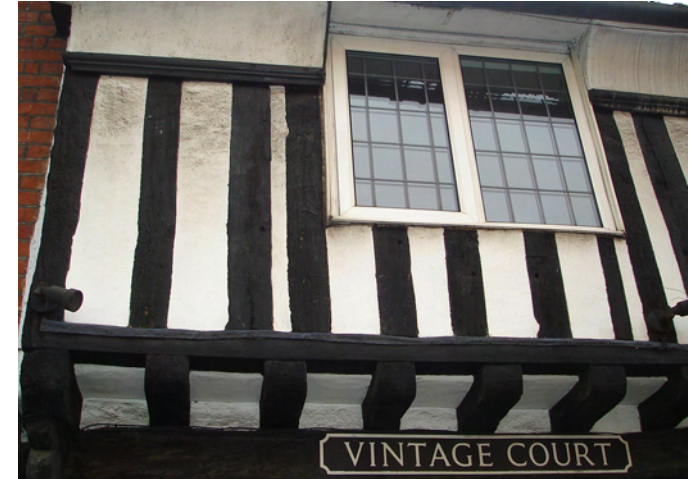
2. Tudor timber frame construction in Baldock town centre.
