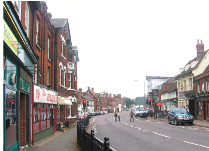
1. Continuous frontages create strong building lines along the gentle curve of Whitehorse Street, Town Centre zone.
