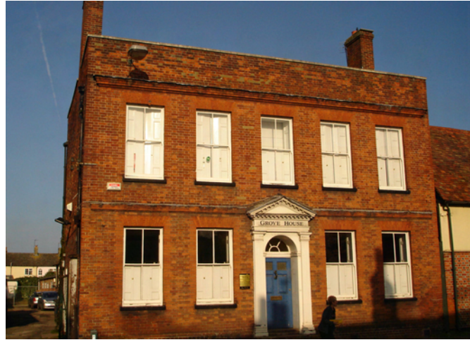
Typical listed Georgian building on Whitehorse Street
