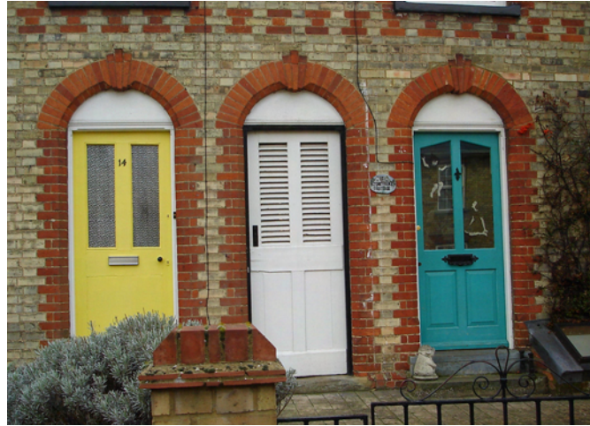
5. Decorative brickwork on residential dwellings at Pembroke Road, Historic High Density zone.
