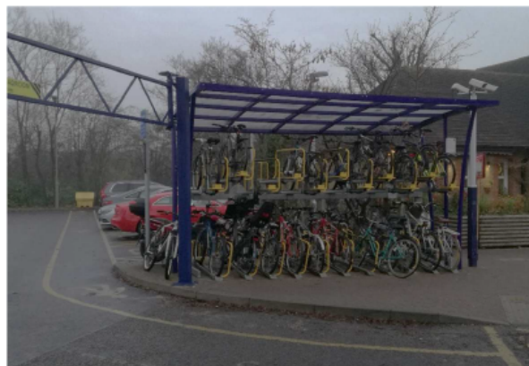
Figure 1: Cycle parking at Letchworth Train Station
