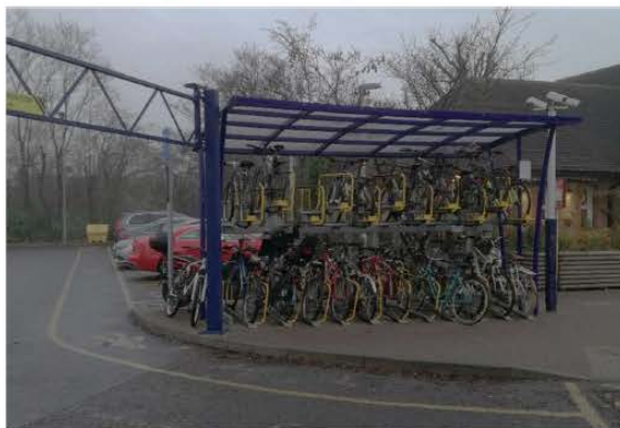
Figure 1: Cycle parking at Letchworth Train Station
