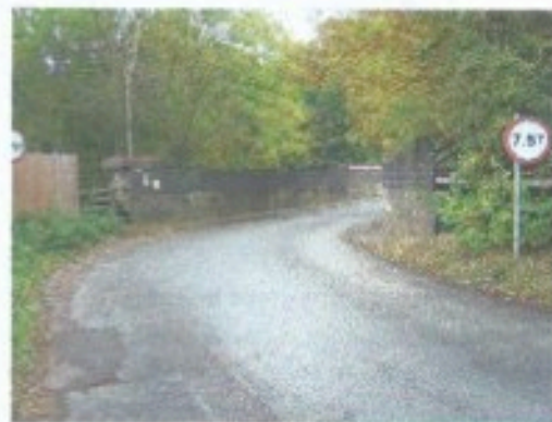
GOLF CLUB BRIDGE
