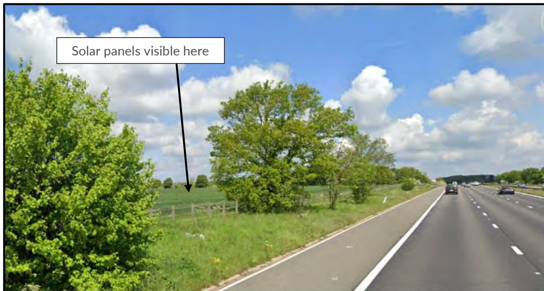
Figure 23 Street view image from location 10 showing the solar panel area
