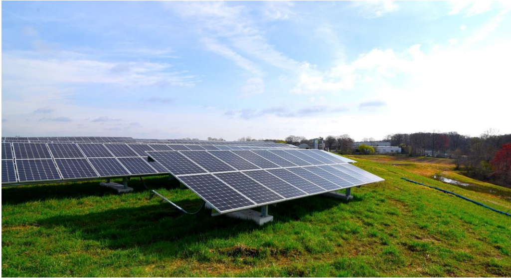
Plate 5.1: Typical ‘No Dig’ Solar Panel Installation
