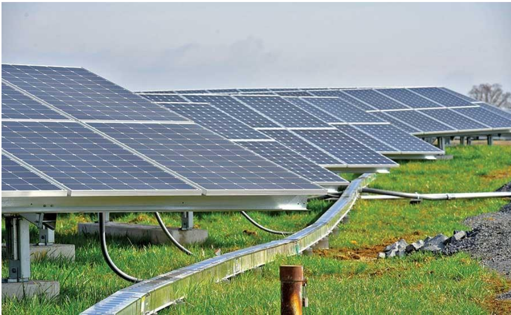
Plate 5.2: Typical ‘No Dig’ Solar Panel and Cabling Installation
