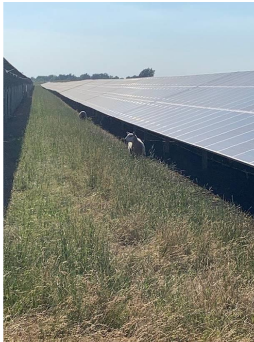
Plate 5.4: Establish Grassland Under Solar Panels
