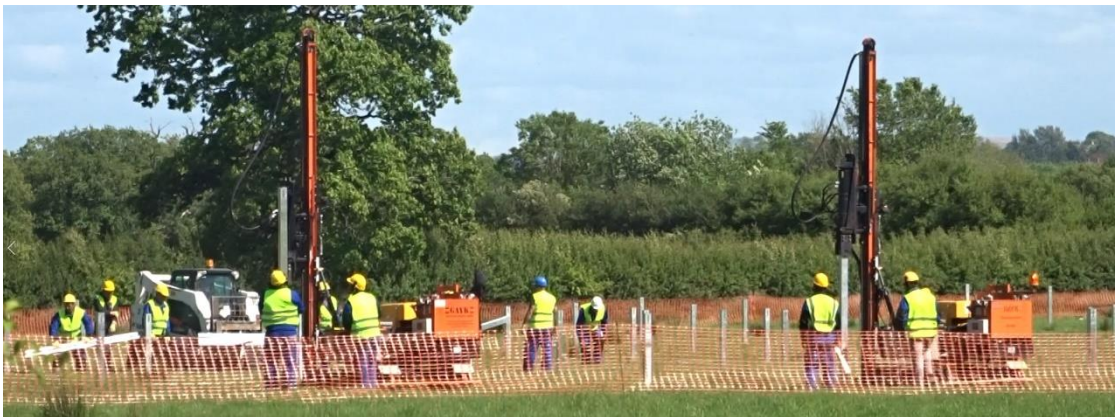
Team Installing Panels
