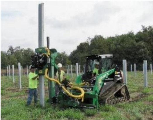
Three Tonne Cabbed Pile Driver and Modern Tractor
