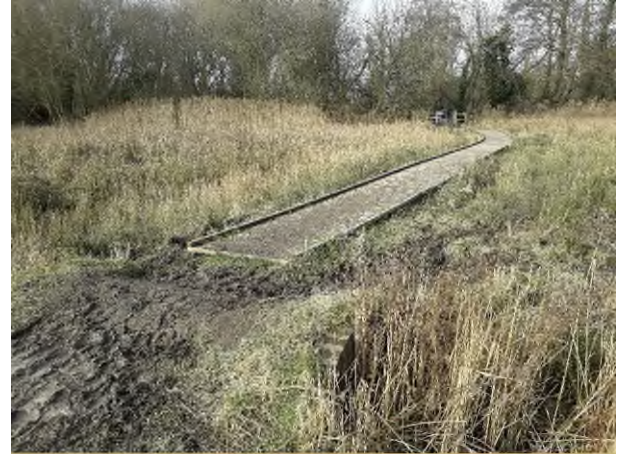
Boardwalk through restored fen
