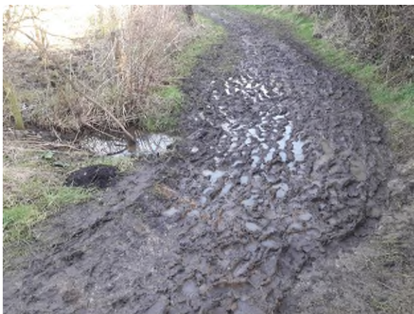
Unsurfaced perimeter path
