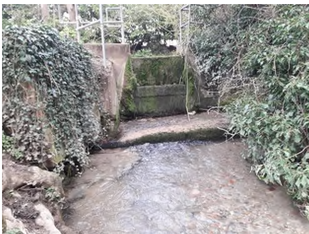
Collapsed weir
