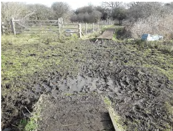
Wet sections between boardwalks
