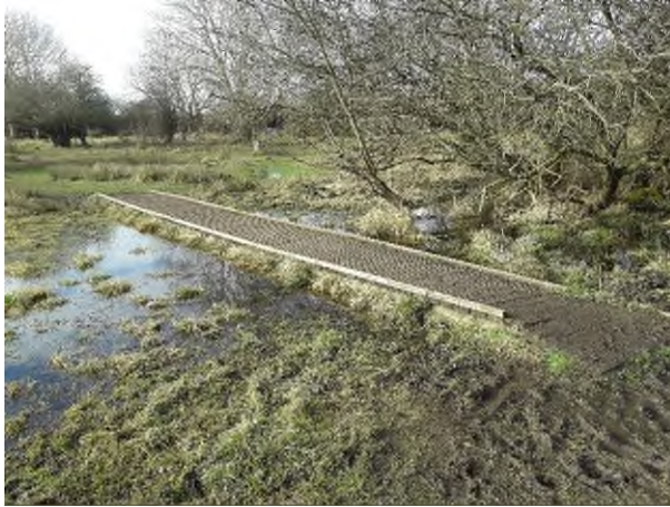
Boardwalk in centre of the site
