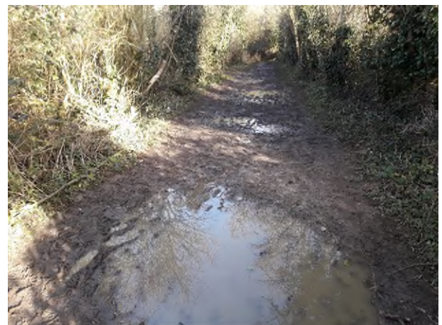
Unsurfaced perimeter path
