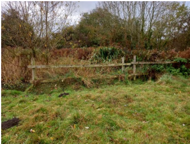
Temporary wooden fencing to protect the riverbank from erosion
