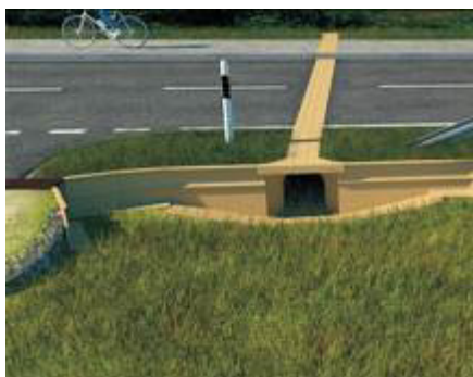
Plates 8 & 9: Examples of under-road badger tunnels, with extended headwalls directing badgers to the tunnel entrance but badger-proof fencing could also be used
